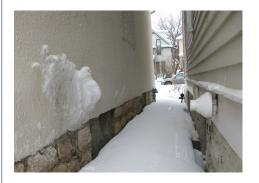
Sidewall vented appliance retrofitted into an older home blows flue gases against the neighbouring house where it has led to ice buildup.
