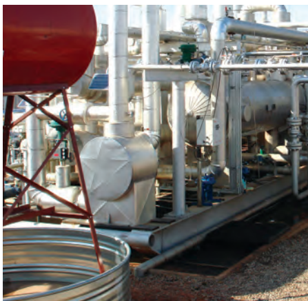
Compact, skid-mounted propane condenser.
