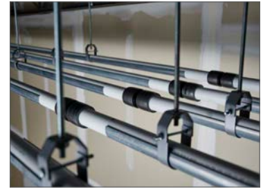
Fig. 5.7: RAUPEX pipe in overhead installation
