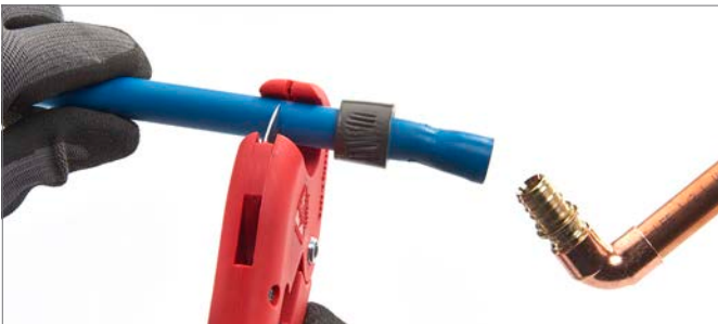
Fig. 4.13: Cut off 3 in. of pipe from end prior to making new joint
