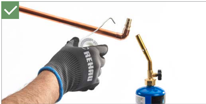
Fig. 6.19: Solder prior to making EVERLOC+ connection
